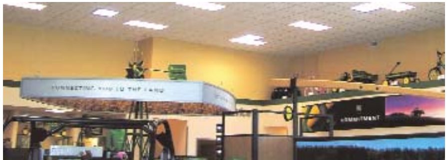
The BTI Greensburg facility uses solar tubes and skylights for much of their lighting.
