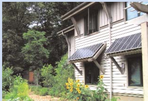
Warren Wilson College's EcoDorm, solar panels are used to shade the interior from the summer sun while fresh fruits and vegetables grow ripe on the vine.
